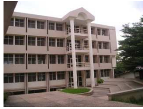
Fig 1 View of the building at CAP, KNUST
