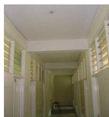
Fig 3 Corridor showing high level windows of the building
